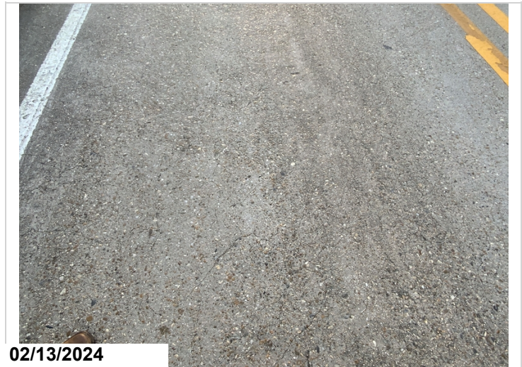
Scattered areas of map cracking.
