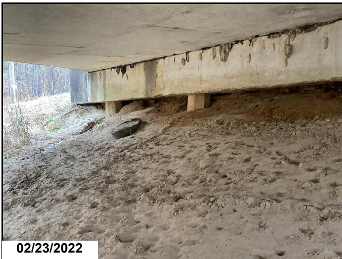
Scour abutment 2 all pile exposed
