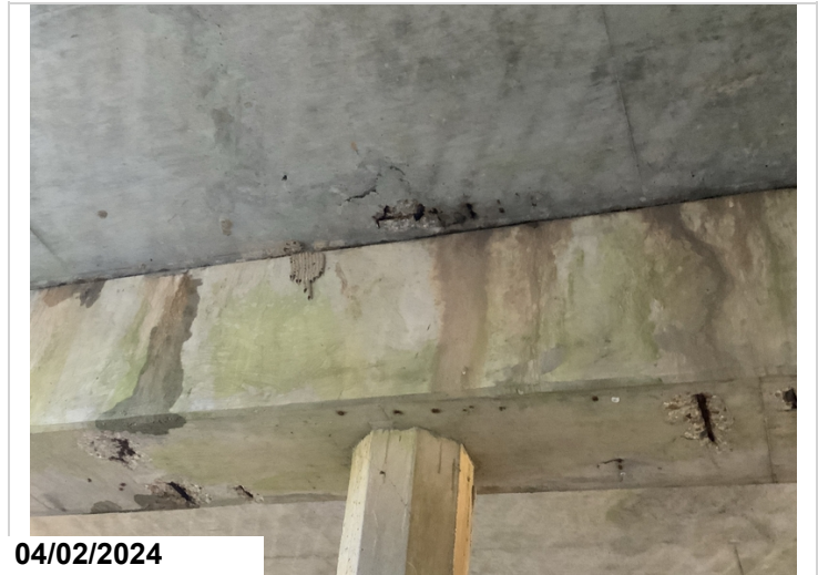
Span 2 soffit exposed rebar ahead of bent 2.
