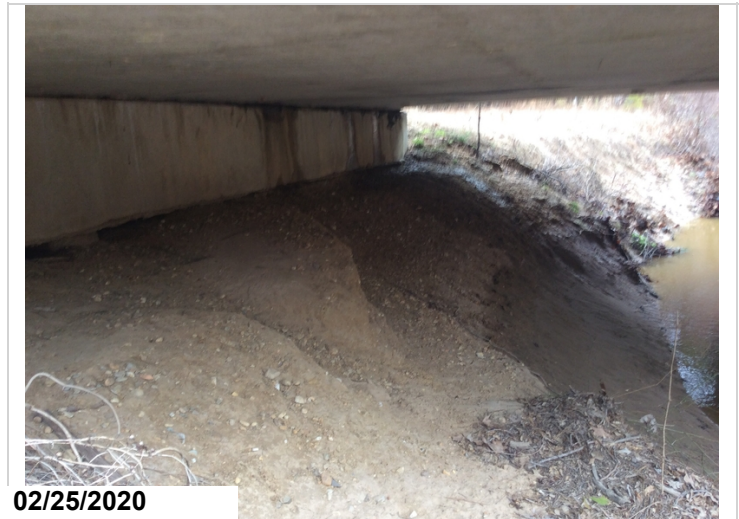
Abutment 1, scour back under abutment cap, and scour encroaching the abutment cap from C/L left.
