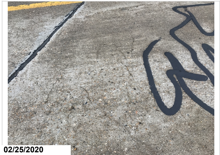
Span 3, map cracks
