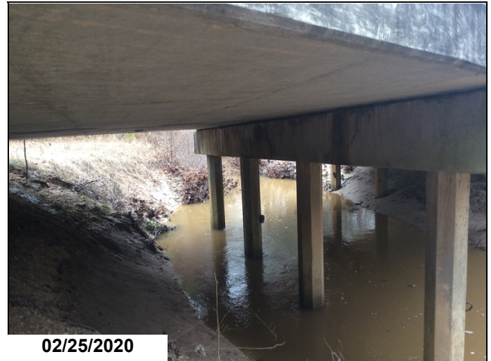
Abutment 1 slope erosion.
