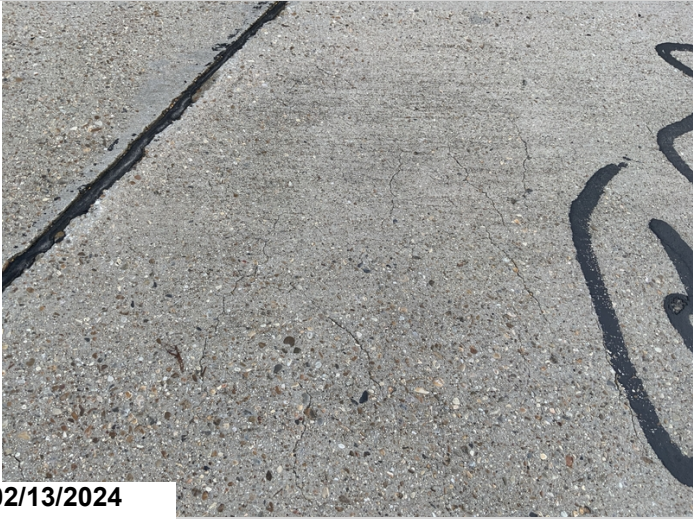
Unsealed cracks span 3 common all spans.
