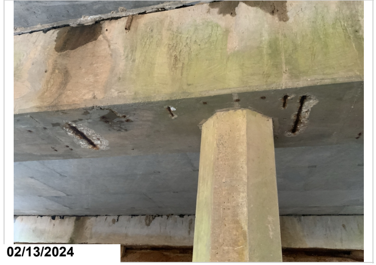
Bent 3 cap bottom exposed rebar, common bent 2.
