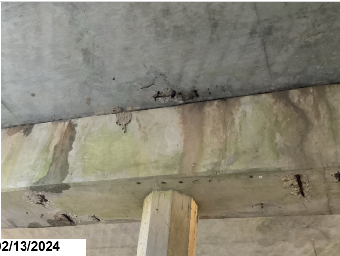
Span 2 soffit exposed rebar ahead of bent 2.
