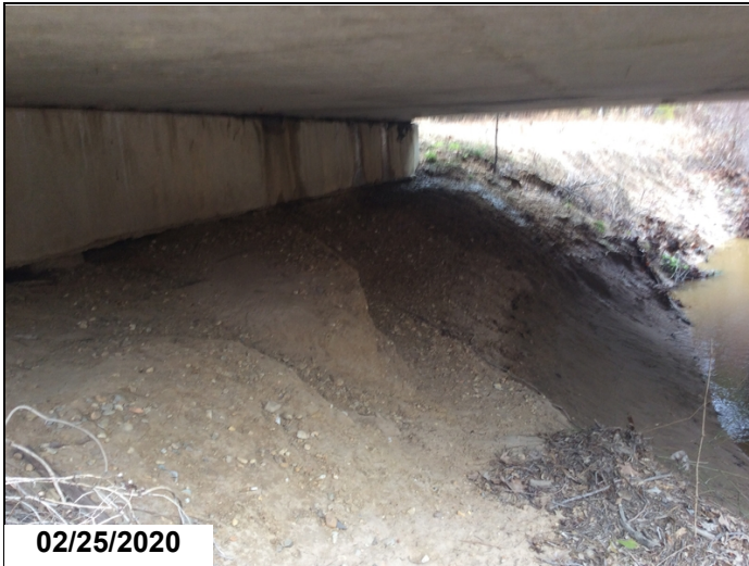
Abutment 1, scour back under abutment cap, and scour encroaching the abutment cap from C/L left.
