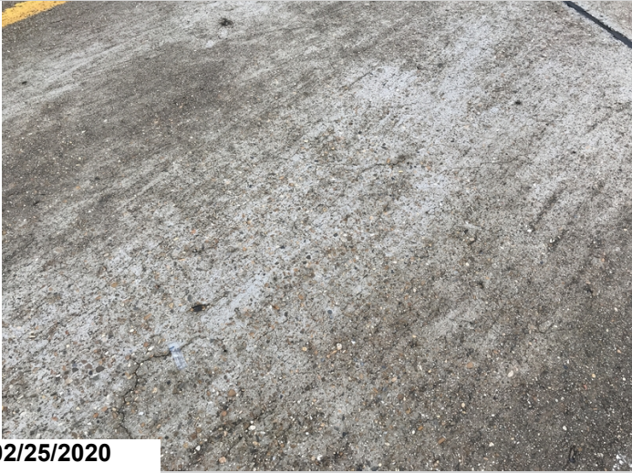
Span 2, map cracks
