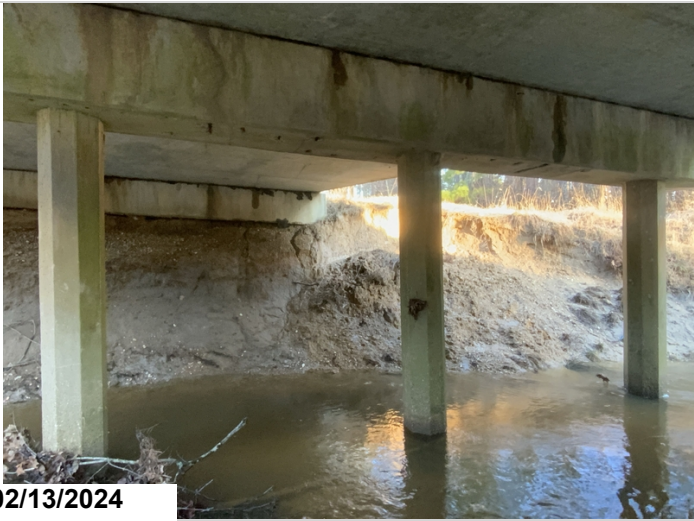
Bank erosion encroaching left side abutment 1.
